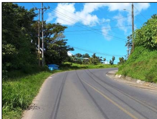
Figura 10. RN N703, sector montañoso
