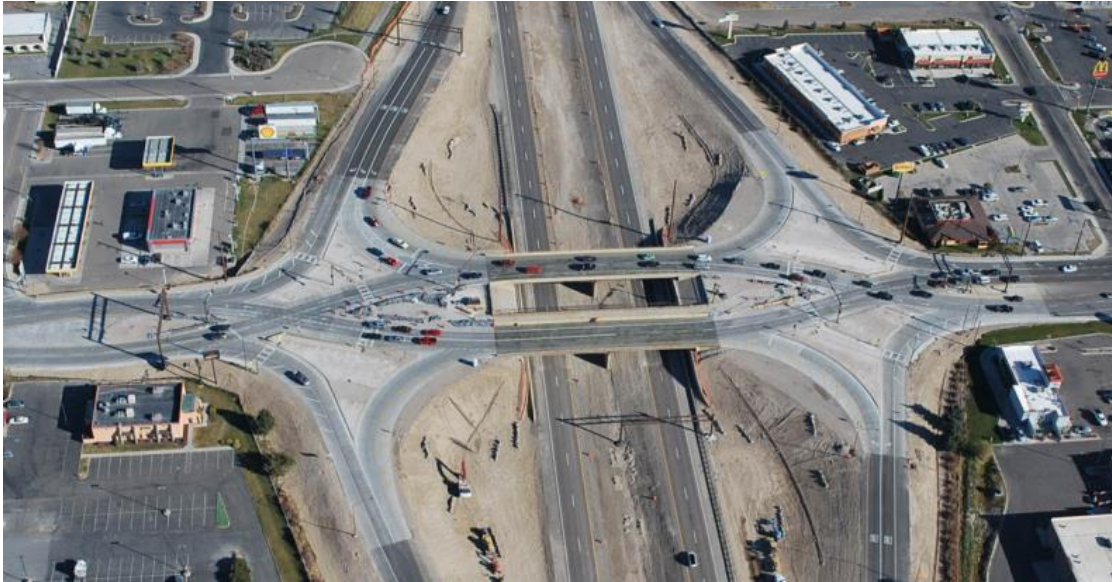
Figura 120. First Constructed DDI In Idaho At Interstate 86 And US 91/Yellowstone Highway
