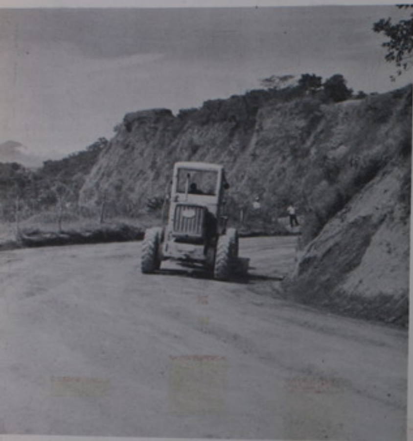
VILLA COLON-PURISCAL RECONSTRUCCION
