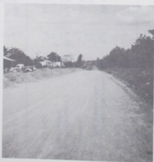
2. CARRETERA ZAPOTE _ CURRIDABAT
