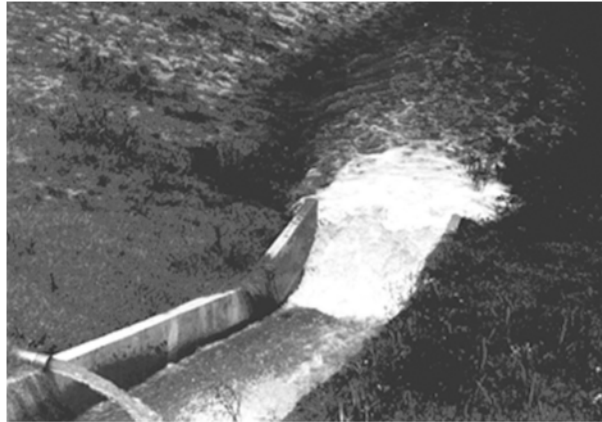
Fig. 6-6 Salida de alcantarilla tipo caja. (AASHTO, 3.5.2 Permanent Erosion and Sediment Control Measures; Chapter 3 - Erosion and Sediment Control in Highway Construction, 2006)
