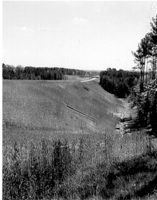
Fig. 6-2 Example of vegetated batter. (AASHTO, 3.5.2 Permanent Erosion and Sediment Control Measures; Chapter 3 - Erosion and Sediment Control in Highway Construction, 2006)
