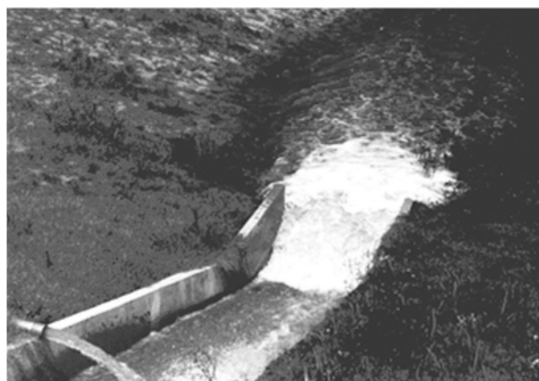
Fig. 6-6 Box culvert type output. (AASHTO, 3.5.2 Permanent Erosion and Sediment Control Measures; Chapter 3 - Erosion and Sediment Control in Highway Construction, 2006)
