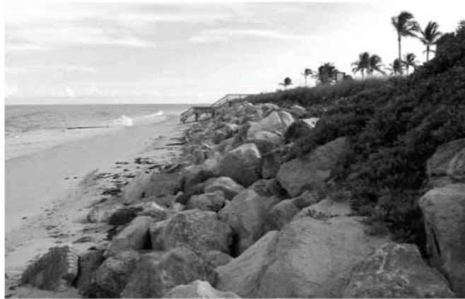
Fig. 6-8 Rock coating. Extracted from (AASHTO, 2006)
