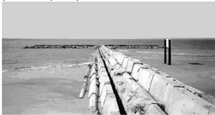
Fig. 6-9 Jetty of concrete pre-built units. Extracted from (AASHTO, 2006)
